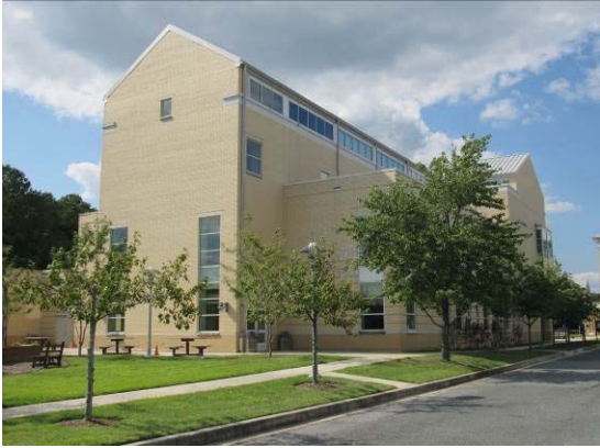
Exterior from Southeast
